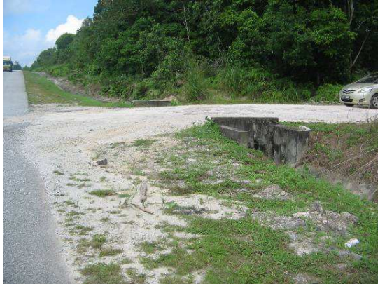
Access road to site (2km)
